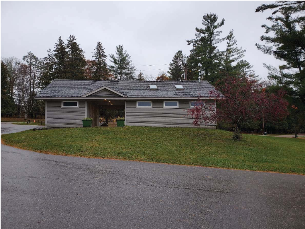
New shower/restroom building
