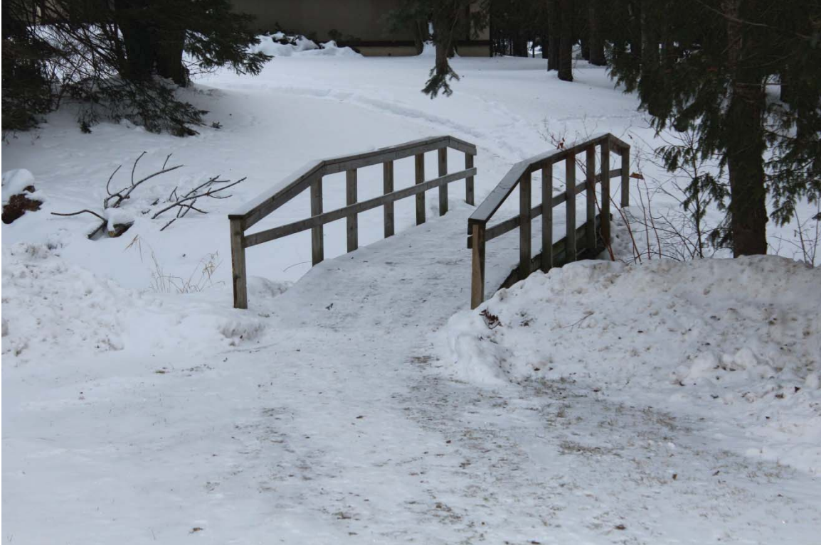
Footbridge at Pineview Park
