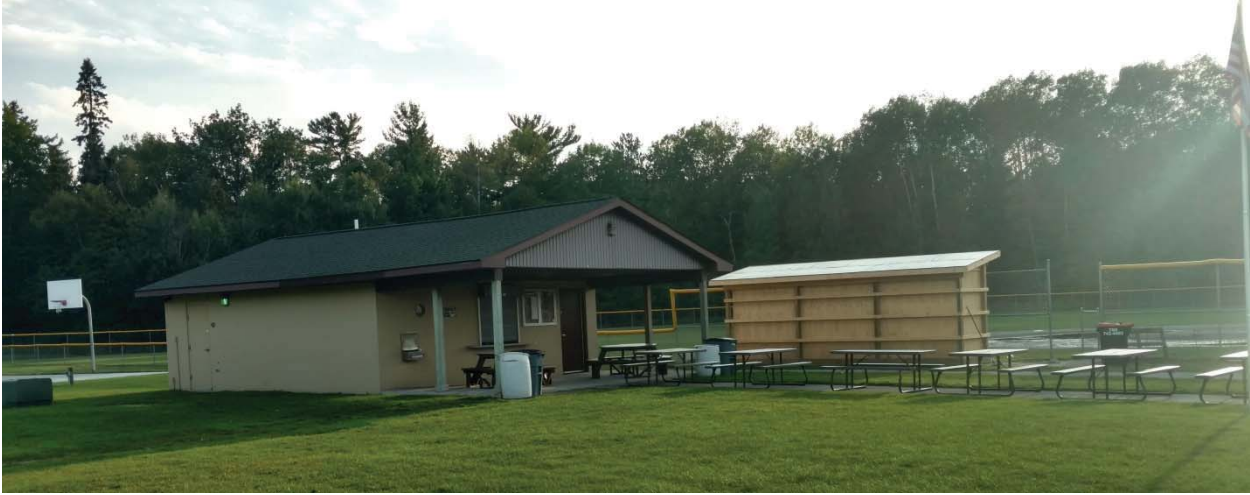
Existing Ballfield Complex (new dugout under construction)
