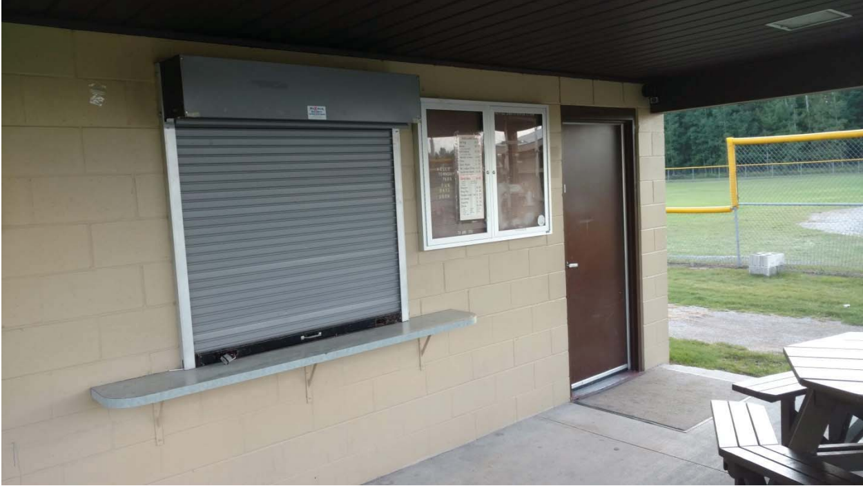
Concessions window on pavilion and restroom building
