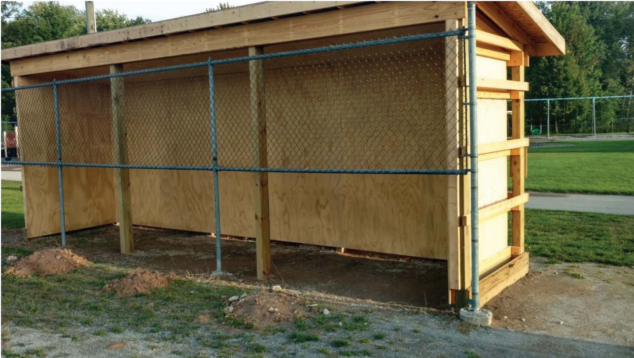
New Dugout under construction
